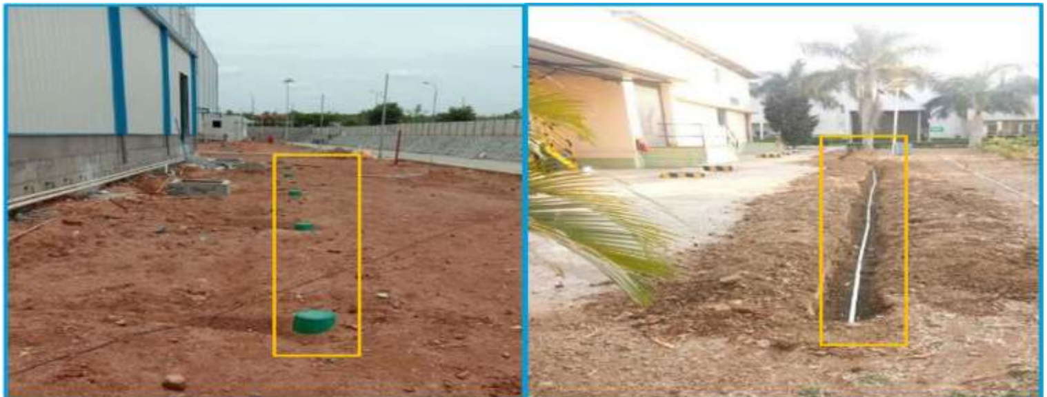
Type A & Type B Earthing Electrode
